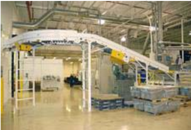
Old Material handling system.
